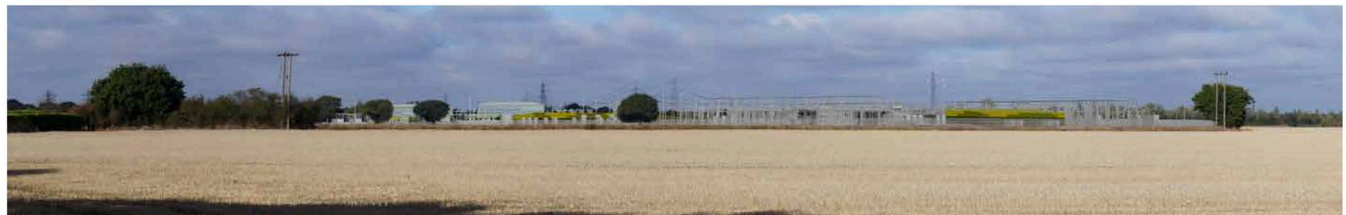
Plate 137 - Indicative photomontage showing both North Falls AIS substation and Five Estuaries GIS substation with transition colour concept - from Ardleigh Road / Jennings' Farm (ES Viewpoint 4)
