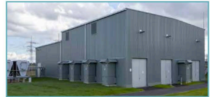
Plate 32 - Typical STATCOM building. Source: https://www.entsoe.eu/technopedia/techsheets/static-synchronous-compensator-statcom/
