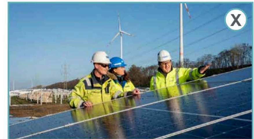
Plate 85 - PV panels. Source: RWE
