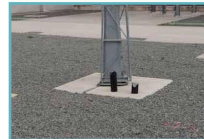
Plate 59 - Concrete pads to base of electrical equipment
