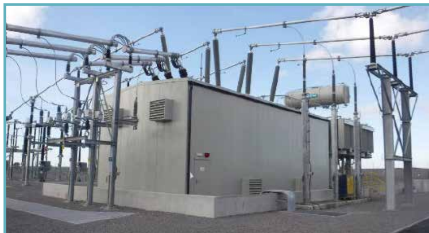
Plate 42 - Transformer with noise enclosure (source - RWE)
