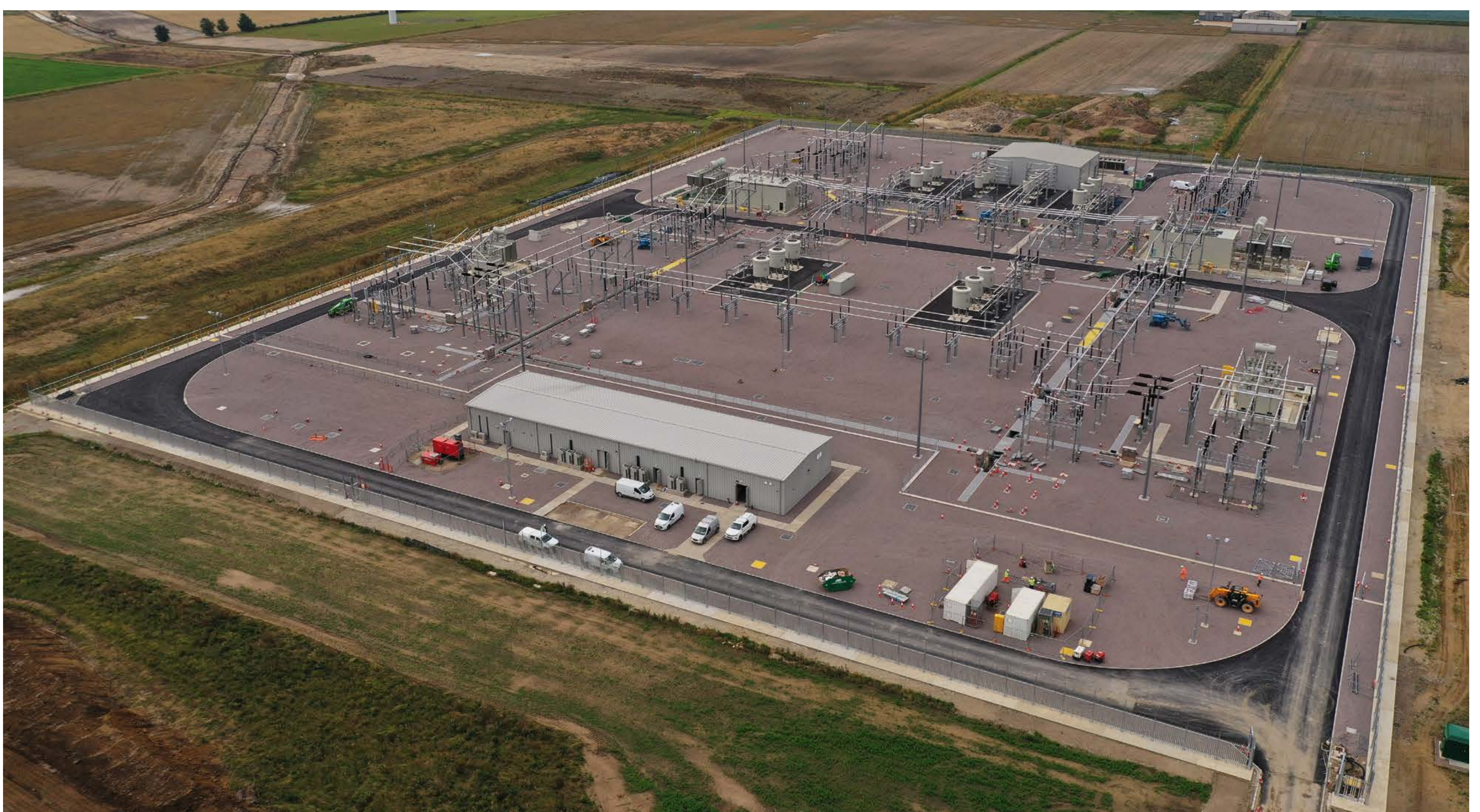
Typical AIS onshore substation (RWE Triton Knoll Offshore Wind Farm)
