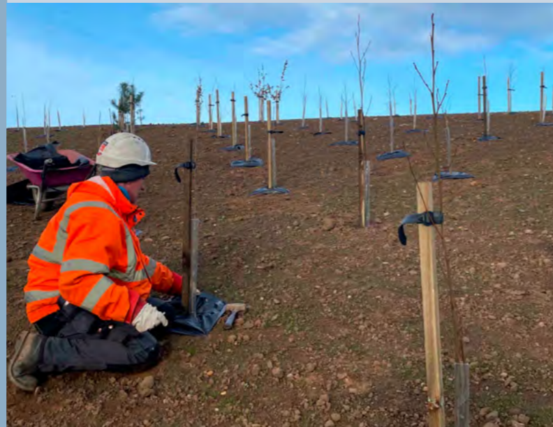
Below: Landscape reinstatement, planting trees following construction works.
