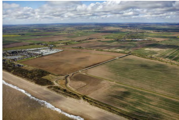
Indicative image of reinstatement. Image courtesy of RWE from the construction of Triton Knoll Offshore Wind Farm, Lincolnshire. North Falls Offshore Wind Farm's reinstatement may differ.
